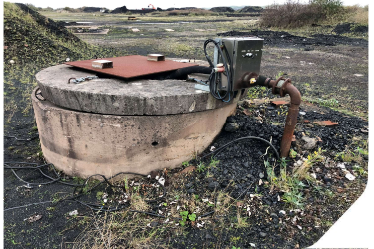
Plate 22: Redundant installation located in the south eastern part of the site
