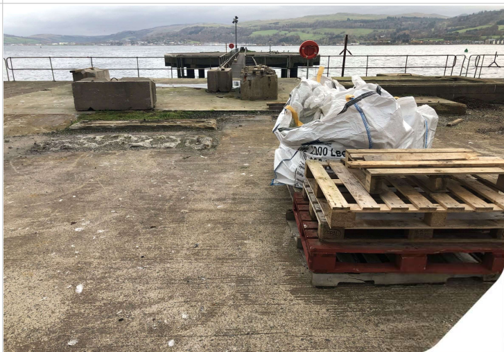
Plate 05: Materials/waste placed on the pier (at the bottom northern end of the pier)
