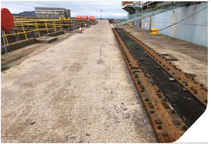
Plate 04: Rail track on the pier facing SW
