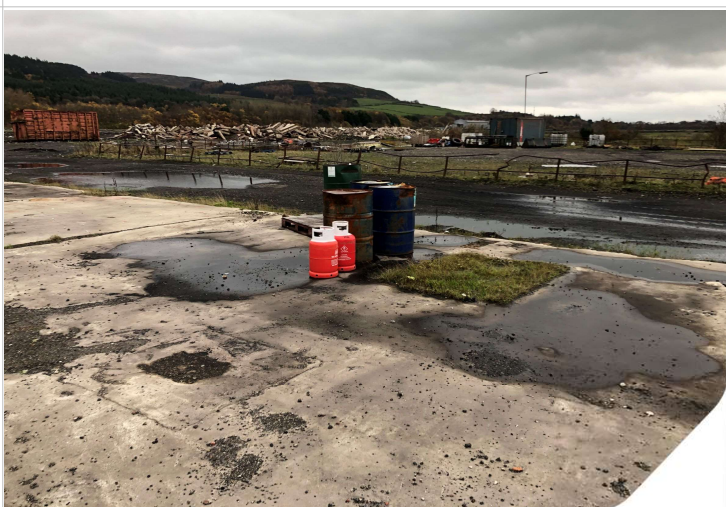
Plate 11: View of site showing drums and gas cylinders facing SE
