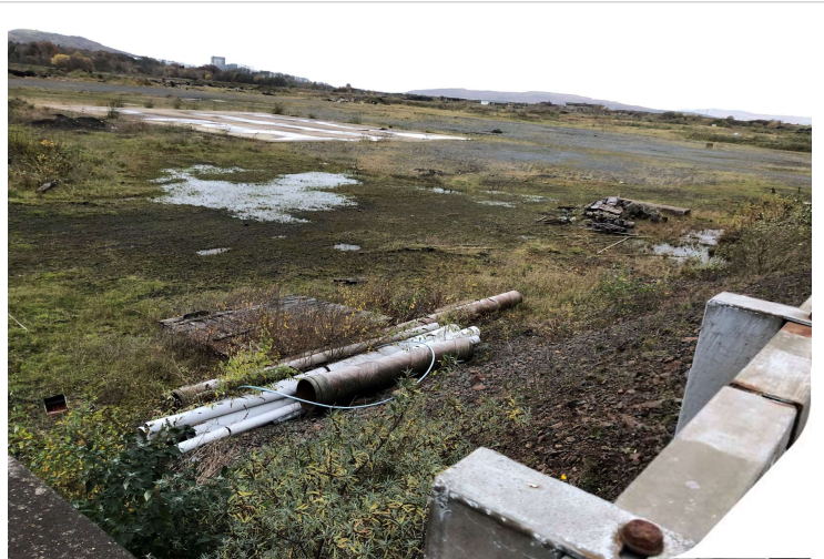
Plate 24: View of the southern part of the site from the bridge facing S and SW
