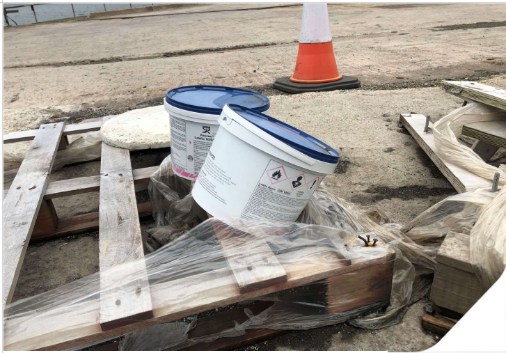
Plate 03: Waste bins and wooden pallets facing NE
