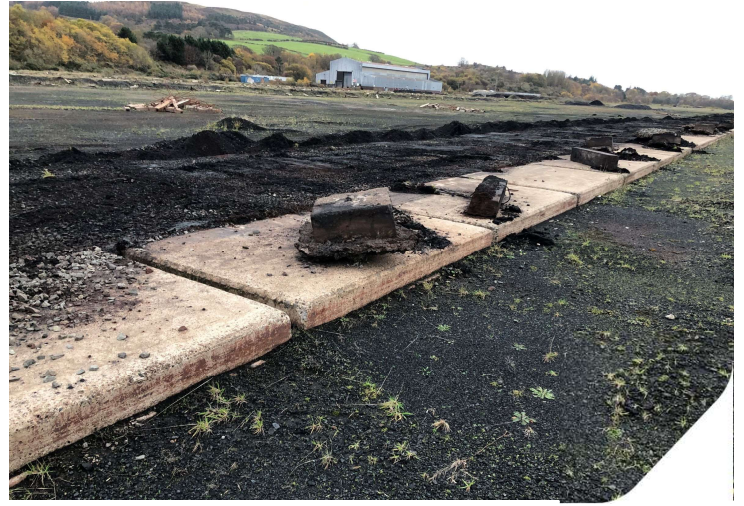
Plate 20: Removal of rail track facing NE
