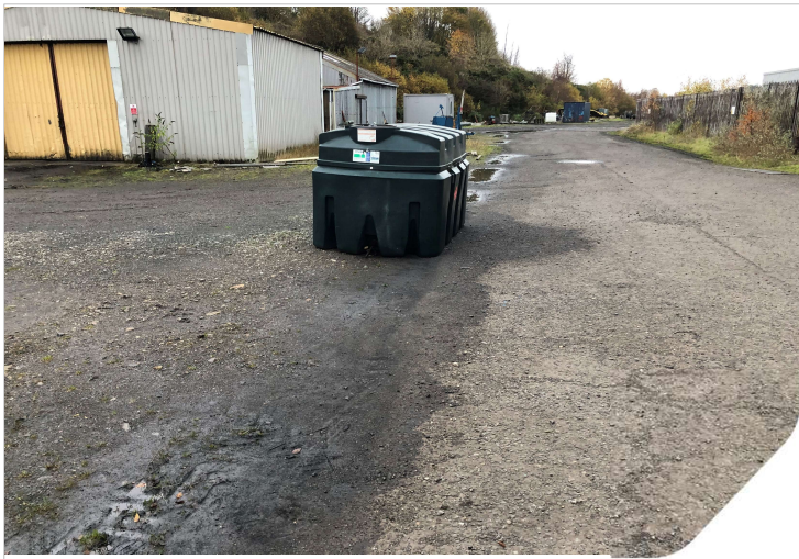
Plate 25: Fuel/oil tank in the yard area. Evidence of oil leak observed (i.e., dark staining on the ground around the tank and the visible oil sheen. Hydrocarbon odour was also noted)
