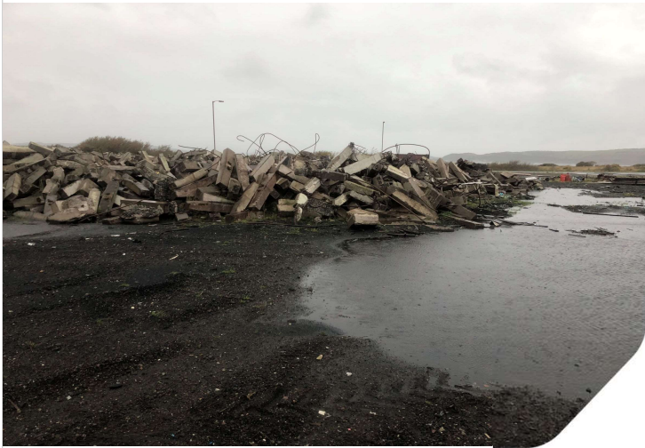
Plate 33: Pile of concrete blocks (removed rail track Footings) facing S
