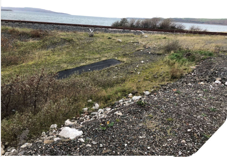
Plate 07: Ground depression in the north western part of the site, with a black fabric at the base of the depression
