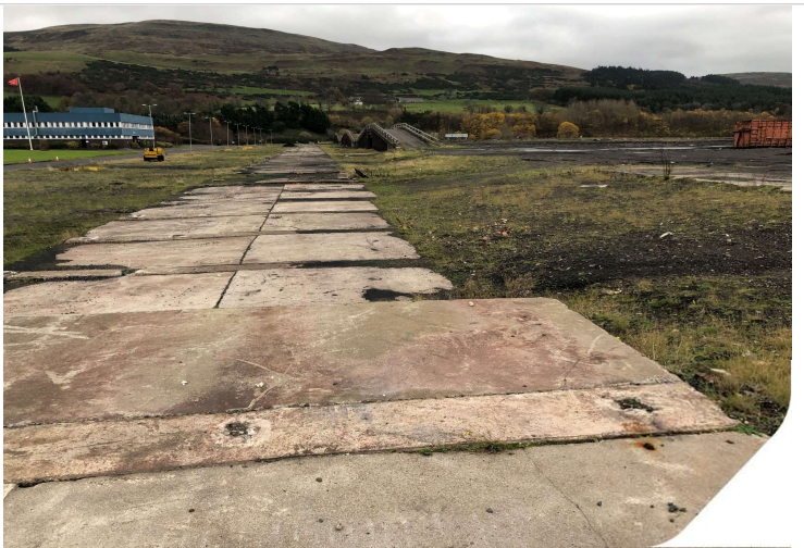
Plate 10: Showing a strip of concrete slab (former conveyor area) facing E
