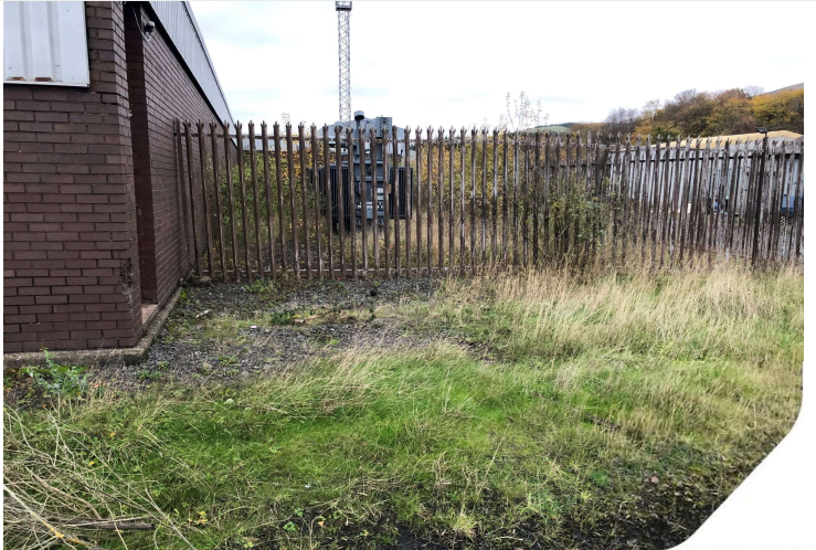
Plate 28: Transformers (sub-station) facing NE
